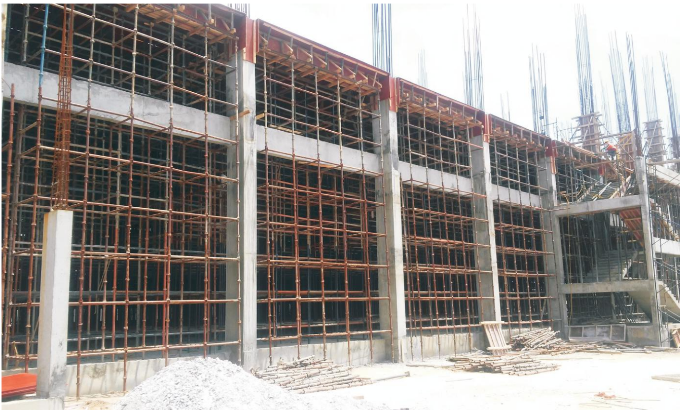
Ashirwad Pipes Warehouse
